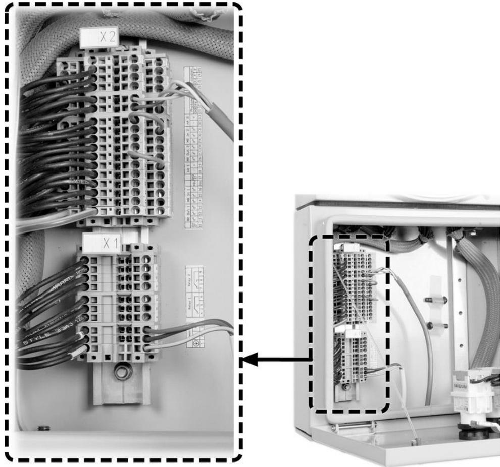
Figure 10: Position of SIREL Ex terminals
