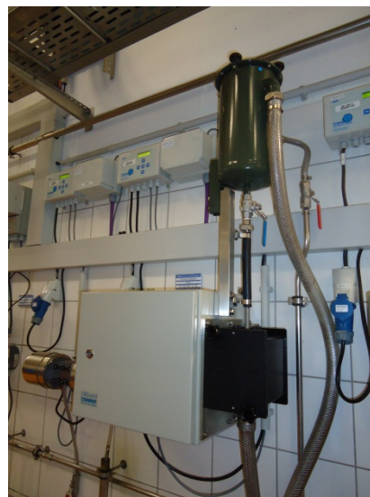
Picture 2: Installation example of an Oil-in-Water Analyzer OilGuard
