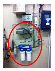
Picture: ColorPlus Bypass in raw water with filtration of sample
